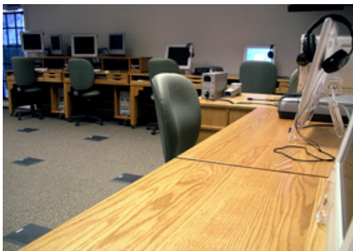
Figure 3. Raised Floor with Network and Electrical Outlets
